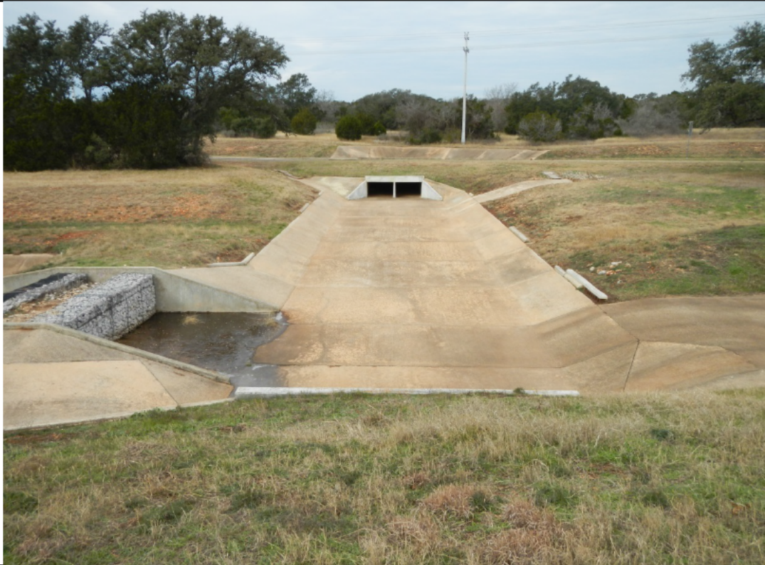
Photograph 7. View of median culvert for Tributary 1 of Danz Creek. View is to the west.
