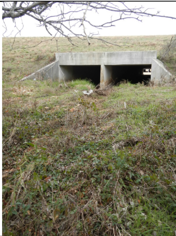
Photograph 8. View of Tributary 1 of Danz Creek. View is to the west of the northbound MoPac lanes.
